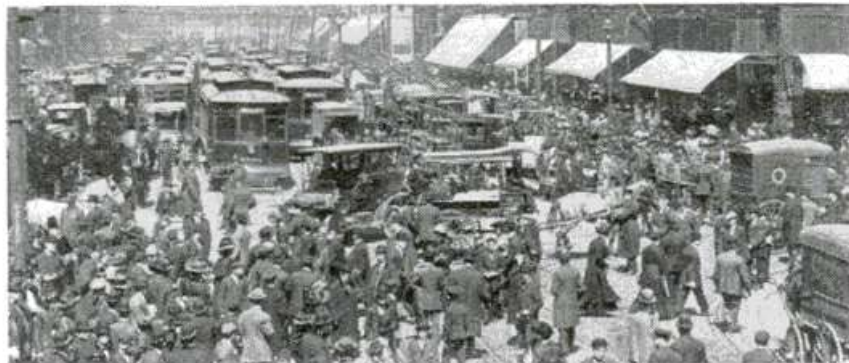
CHICAGO'S BUSY CENTER WHERE ROTARIAN WHITTLE SAW DANGER TO THOUSANDS DAILY.
